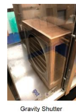
Fig. 4 – Recirculation prevention
