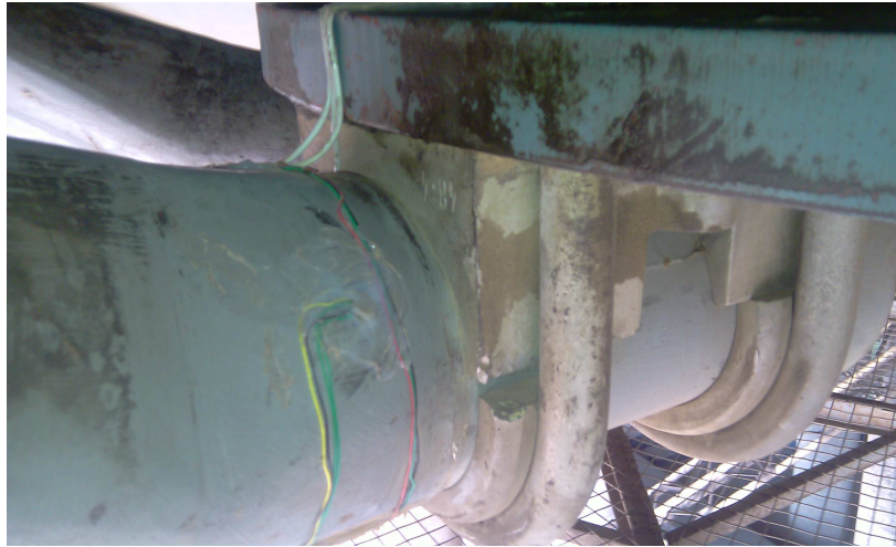
Figure 3: Strain gauge placement on fan blade
